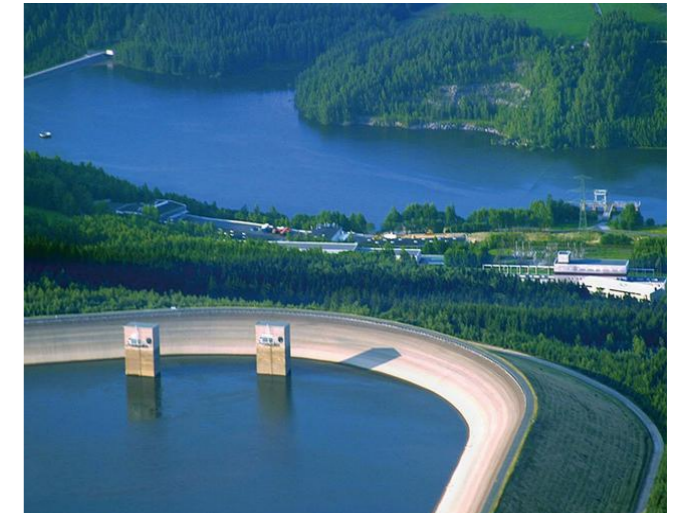
Project name: Markerbach Pumped Storage Solar Power and Hydropower Plant in Saxony, Germany Project capacity: 4.3 MW
