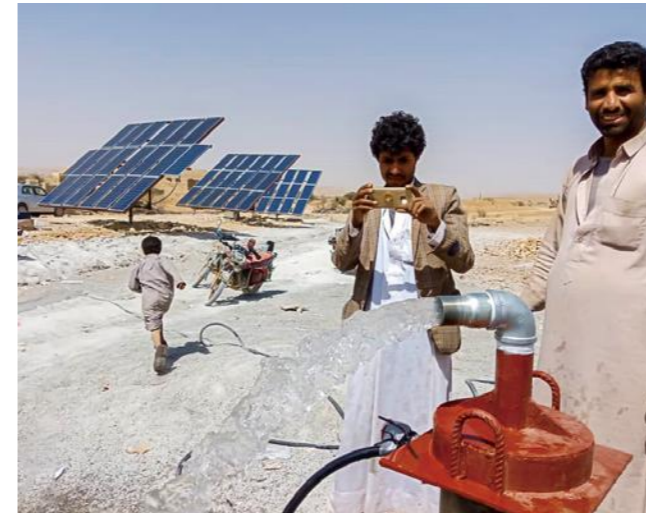
Project name: Solar Power Water Pumping and Irrigation Project in Yemen Project capacity: 10 MW
