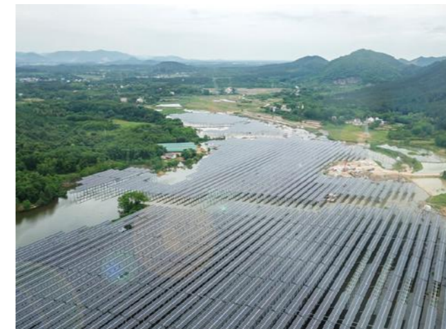
Project name: Solar Powered Fishery Combination Project in Qingyang County, Chizhou Project capacity: 10 MW
