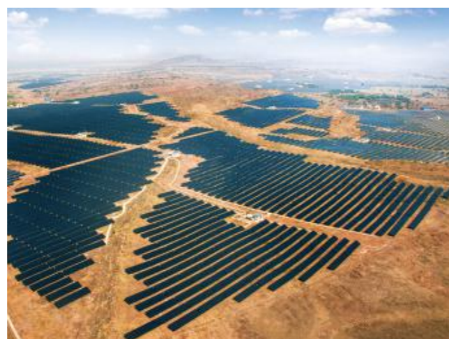
Project name: Solar Power Plant in Bhadla, India Project capacity: 300 MW (196.25 MW out of Suntech supplies)
