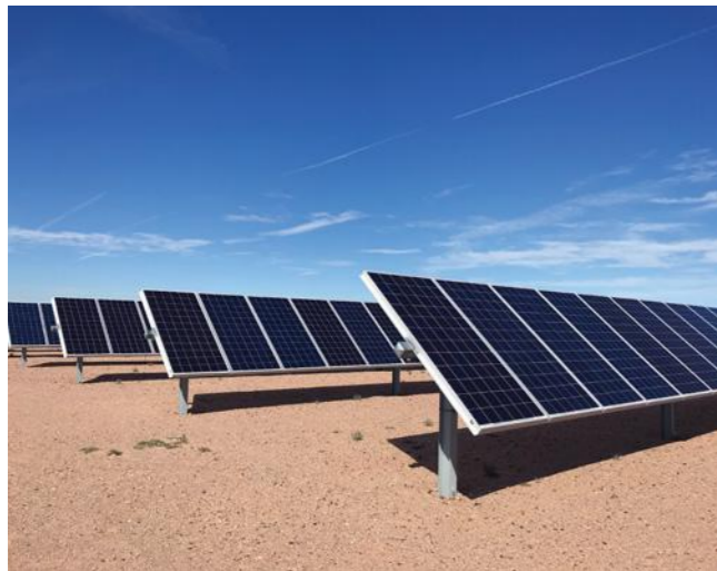
Project name: Solar Power Plant in Oberwesterwaldbahn, Germany Project capacity: 10 MW
