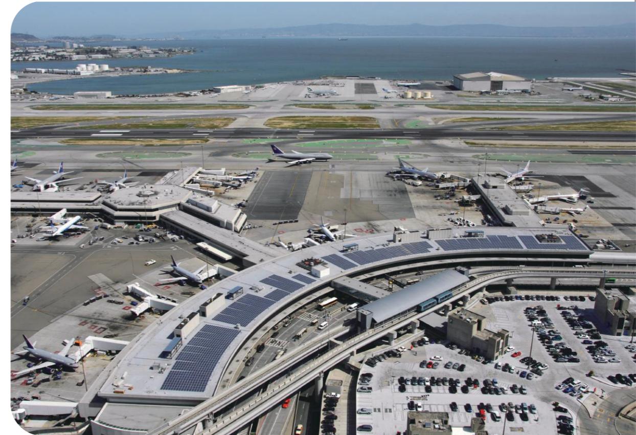
San Francisco International Airport Terminal 3 Rooftop Project
